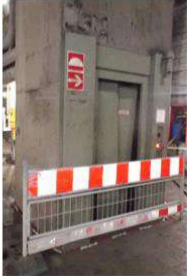
Elevator door pressed in
